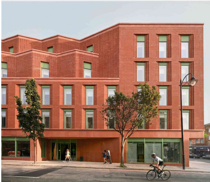
▲ 2.2.e A consistent arrangement of windows and details along vertical and horizontal lines, are also organised into a clear bottom-middle-top hierarchy that creates a highly cohesive and appealing façade.
