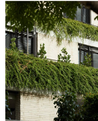
▲ 2.2.l Vegetation is incorporated into the design of this façade, cascading over balconies and emphasising the horizontal ordering of the façade.
