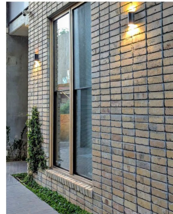
▲ 2.2.i Lighting directed up and down produces diffuse reflections from the building façade which gently illuminates pedestrian areas while limiting glare.
