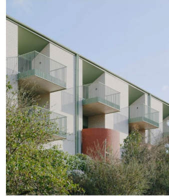
▲ 2.2.h Semi-projecting balconies align with the building's vertical articulation, with green accents cohesively applied to soffits, balconies and downpipes.
