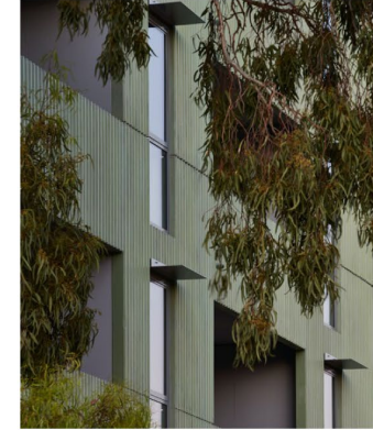
▲ 2.2.j Textured and coloured concrete panels blend in with the surrounding vegetation, and provides a clear ordering of the façade openings, with clean lines reinforced by the discrete detailing at the joints and simple window shades.
