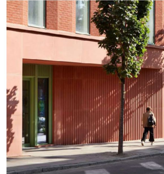
▲ 2.4.b The recessed entry with a fine-grain textured wall, and a colour-accented doorway identifies the building's entry point, while providing amenity and visual interest.
